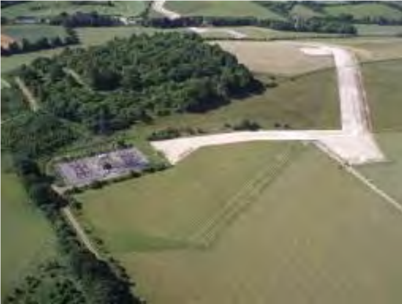
Figure 24 – Moulsoford Down 400kV SEC near Goring
