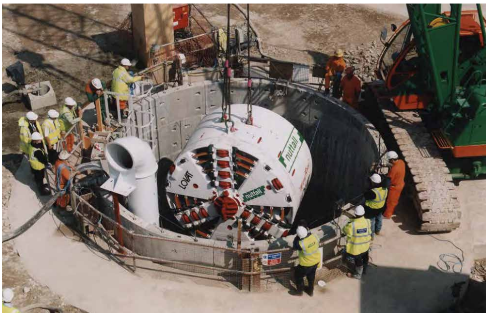
Figure 68 – Head-section of TBM being lowered into working shaft
