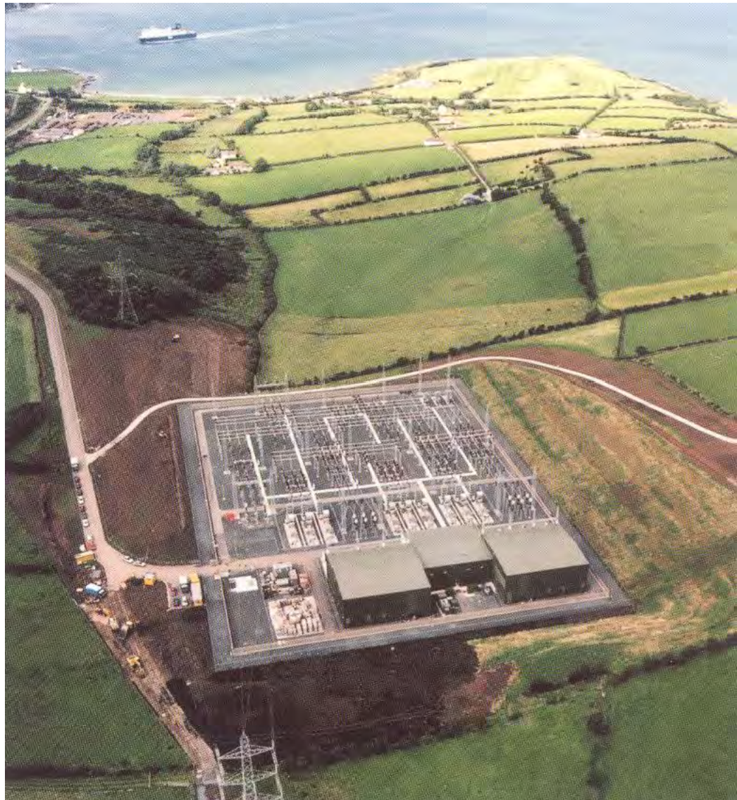
Figure 58 – Ballycronan More 500MW CSC converter station
