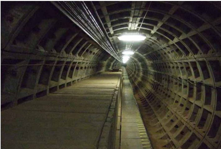
Figure 45 – Wimbledon–New Cross cable tunnel
