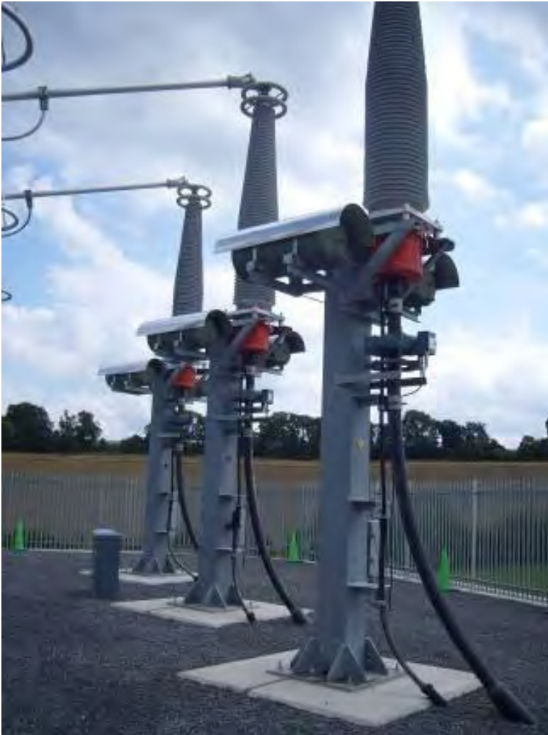
Figure 22 – 400kV terminations installed near Goring
