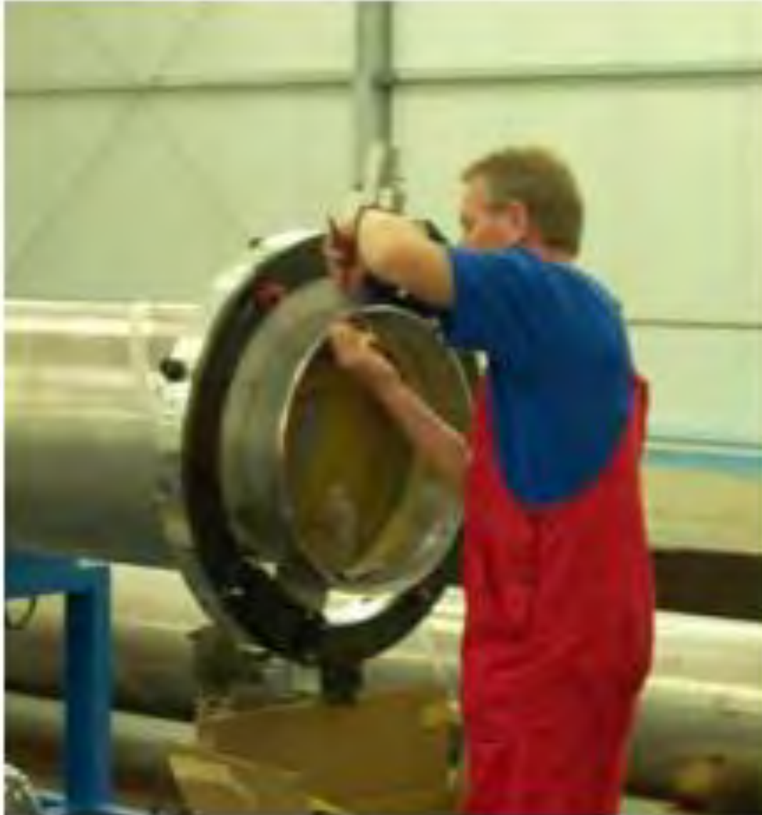
Figure 61 – GIL weld edge preparation prior to connection
