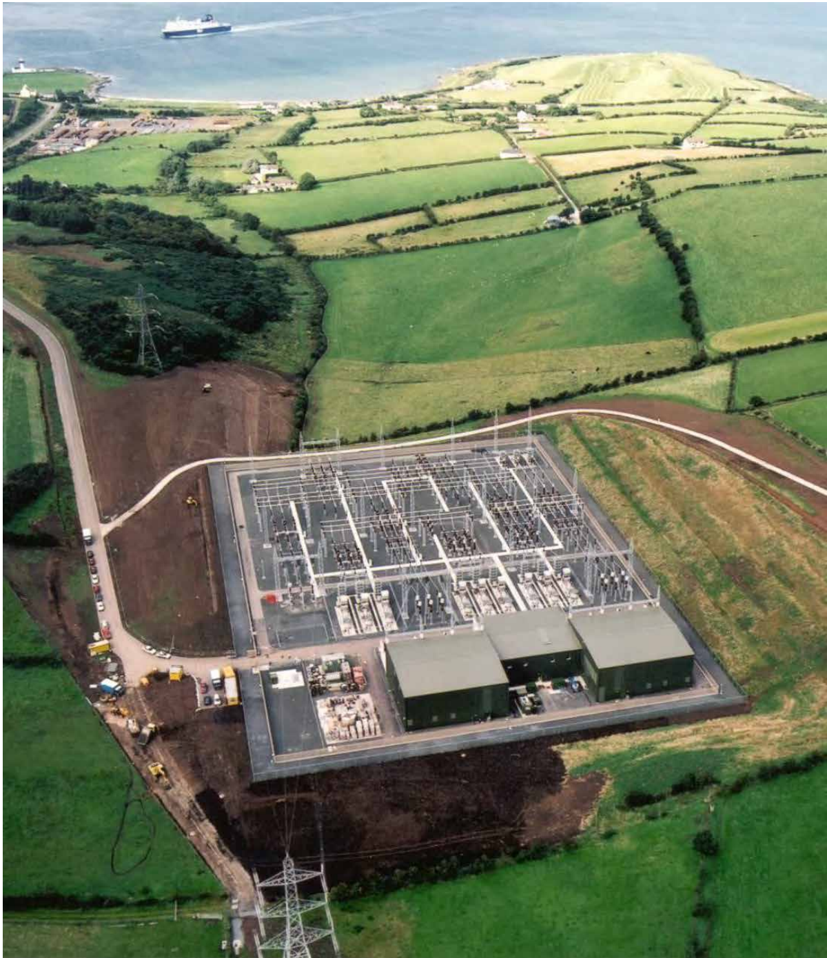
Figure 5 – Ballycronan More 500MW CSC converter station
