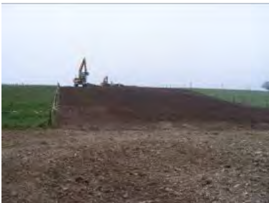
Figure 44 – Topsoil replacement
