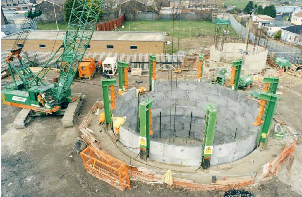
Figure 67 – Hydraulic jacks on caisson technique shaft construction
