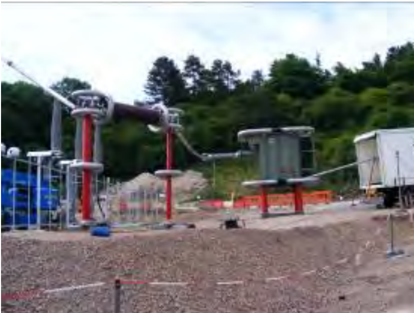
Figure 26 – Cable AC test voltage equipment
