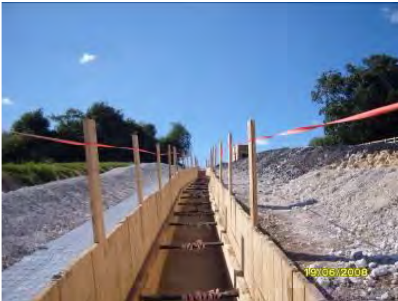
Figure 37 – A close-timbered cable trench
