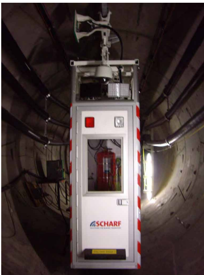
Figure 70 – Tunnel vehicle suspended from monorail
