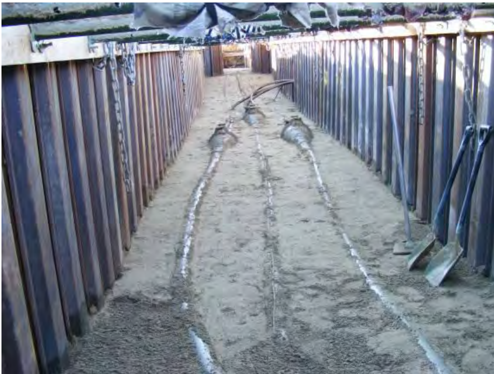
Figure 19 – EHV joint bay containing three Joints
